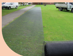
Mesh laid onto existing surface
