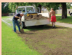
Topsoil brushed over surface
