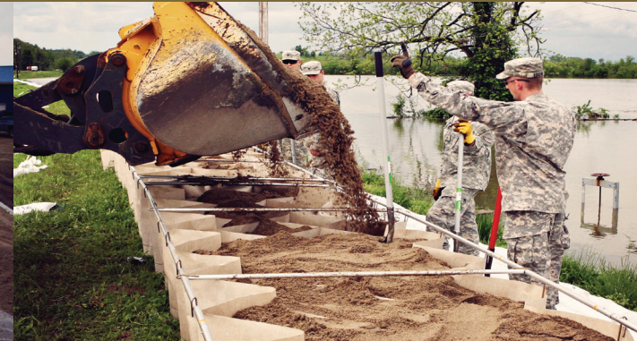
Smithland, Kentucky | National Guard installs Defencell™ on the Ohio and Cumberland Rivers
